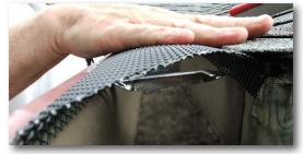
4. Push down screen after it is snapped in to ensure screen is fully expanded and lock into place.
