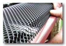
3. Snap the balance of the screen into place.
