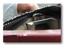
1. Slip the back of the screen underneath the shingles so that it rests on top of the hidden gutter hangers
