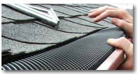
5. Repeat with the next piece, overlapping each section to the full depth of the pre-cut notch.
